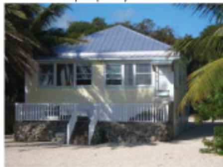
256 Tarpon Street Façade Facing West
