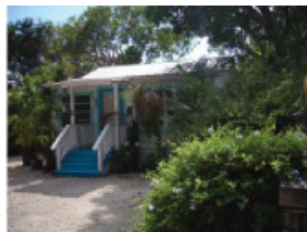
124 Lowe Street Facing South
