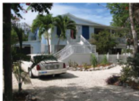
189 Beach Road Facing Northeast
