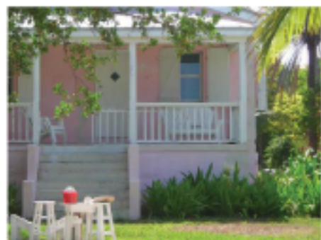
1 Ballast Trail Facing East
