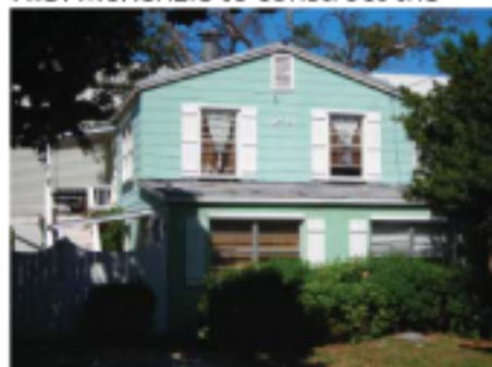
128 Tavern Drive Facing North of Northwest
