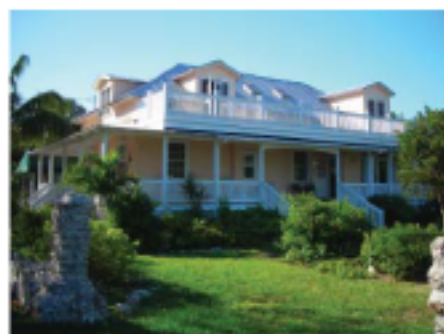
200 Beach Road Facing Northwest
