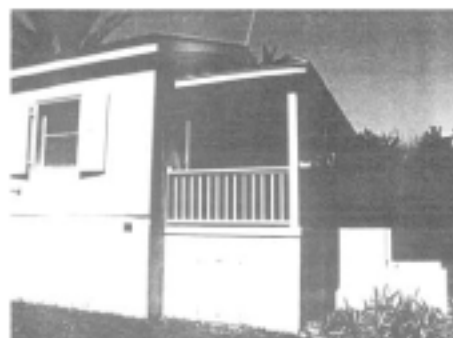
Alice Lowe House circa 1935 Facing Southwest
