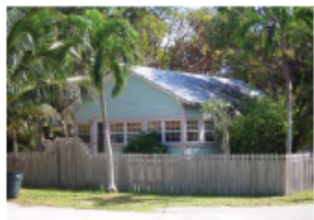
180 Lowe Street Facing Southeast
