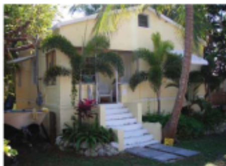
Façade of 192 (current) Lowe Street Facing Southwest
