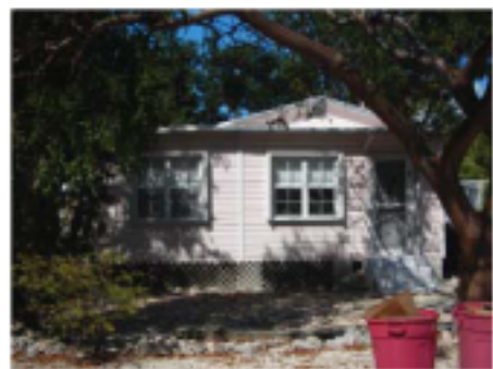
Façade of 185 Lowe Street Facing North
