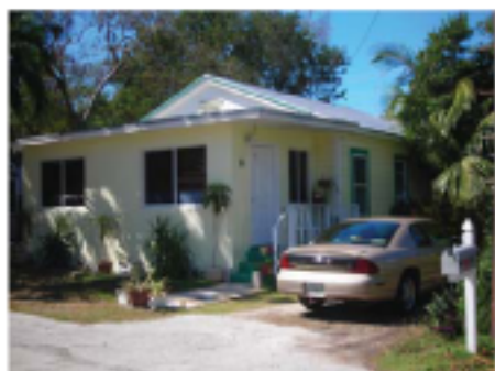
136 Tavern Drive Facing West
