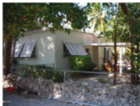
195 Lowe Street Facing North
