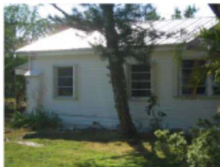
240 Lincoln Avenue Facing Southwest
