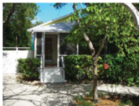
157 Lowe Street Facing Northeast
