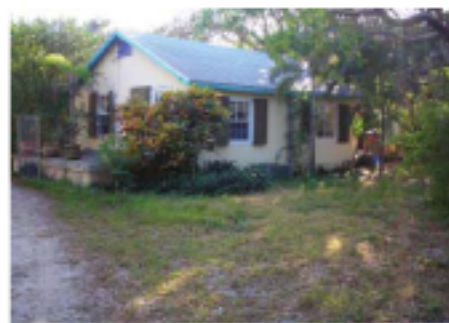
178 Beach Road Facing Northwest.
