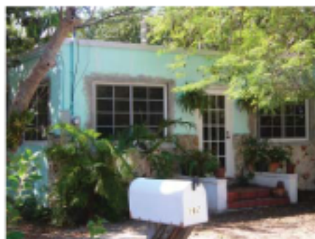
162 Sunrise Drive Façade Facing South
