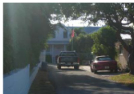
Rodney Albury House Façade Facing East
