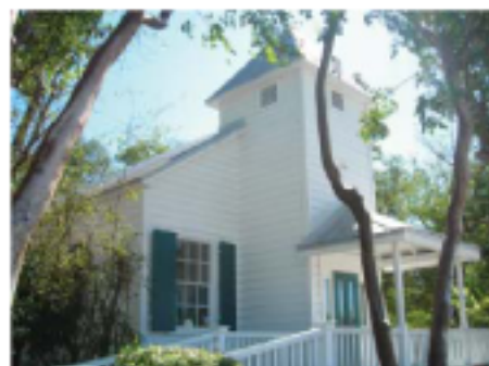
91701 Overseas Highway Facing South
