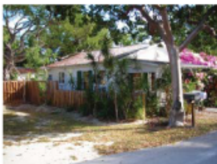
131 Ocean View Drive Main Dwelling Facing Northeast
